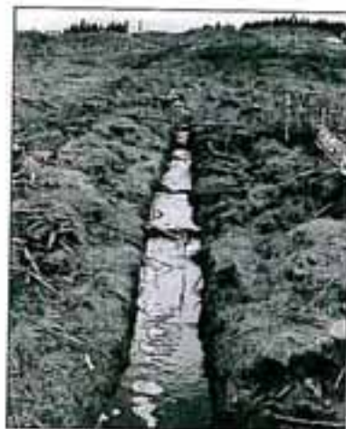
Drains will be blocked using recycled plastic piling
