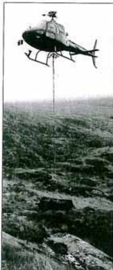
Airlifting railway sleepers for the board walk
