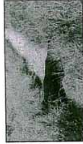
A plastic dam in a bog drain at one of the project sites
