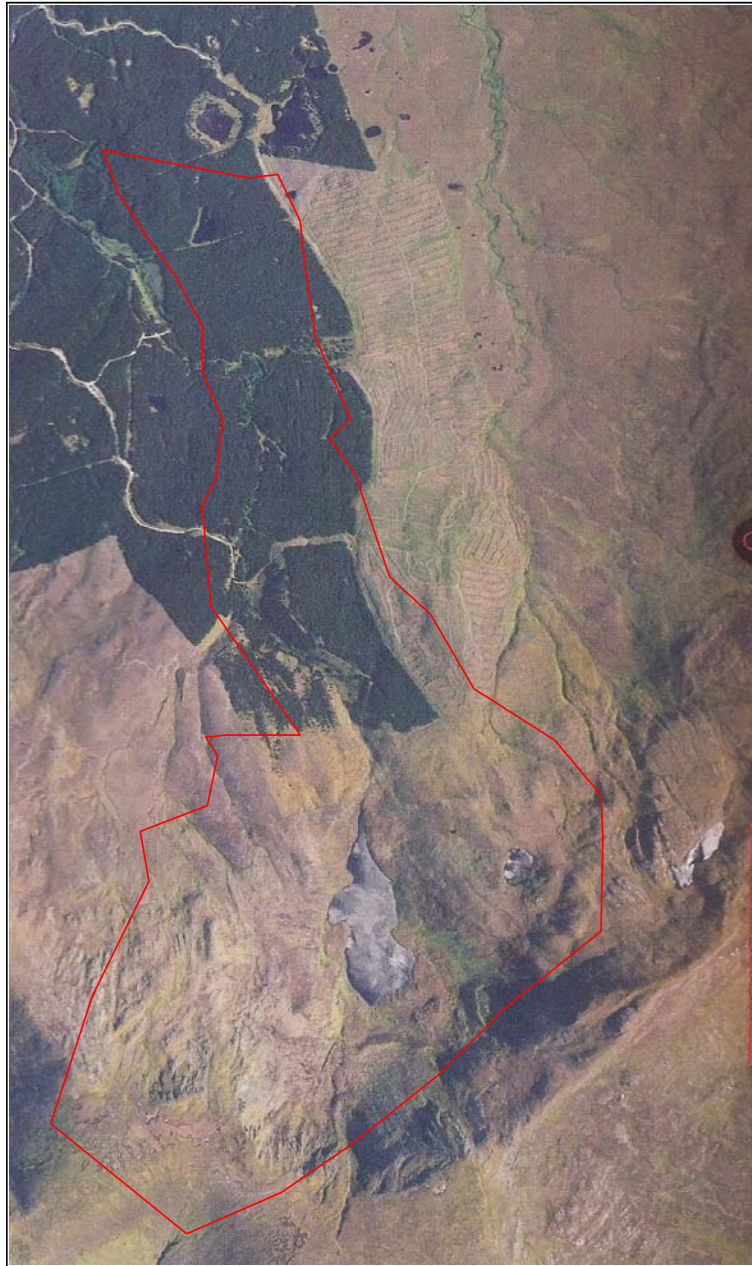
An aerial photograph of the Bellaveeny site at the end of the restoration project. The site outline is indicated in red. Photograph taken in the year 2006.
