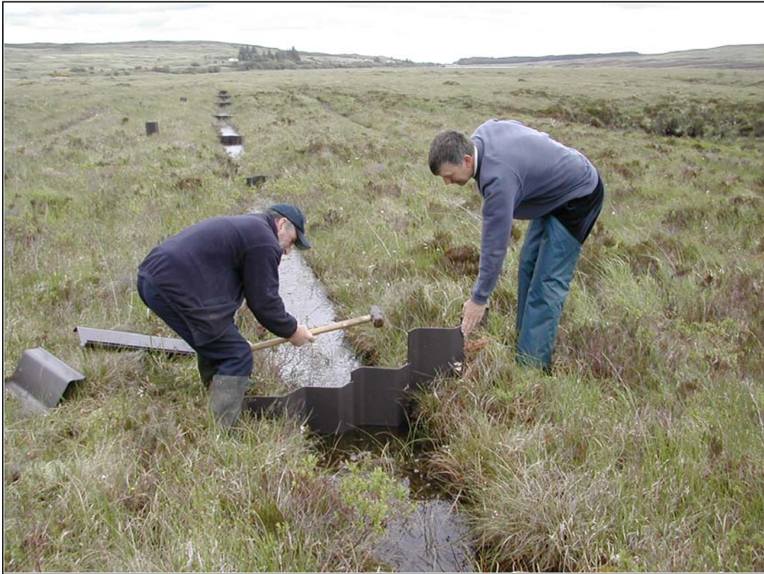
Drains were blocked during 2003/2004 using plastic piling dams.
