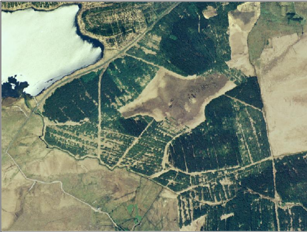
An aerial photograph of the Pollagoona site prior to restoration work taking place. Aerial photograph taken in the year 2000.
