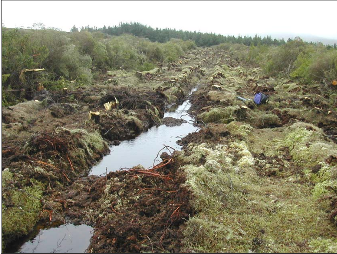
A view of windrowed conifer crop with a peat dam in place. It was generally difficult to put good dams in this site due to the well developed root systems of trees. Photograph taken October 2003.
